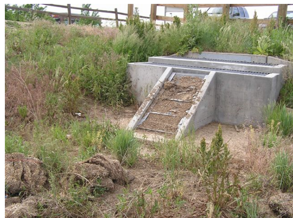
Photos 21 and 22 show before and after construction photos show how straw bales left on site can clog outlet structures later.
