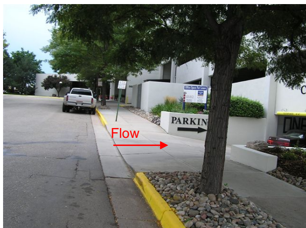
Photo 7. Drainage flows into parking garage due to low curb and sidewalk.
