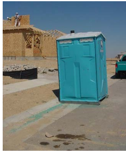
Photo 26. Construction site stormwater management involves many pollutants in addition to sediment, including chemicals and materials used on construction sites, trash and lesser-known pollutants such as biocide (pictured in gutter from portable toilet). Portable toilets and other potential sources of pollutants should be distanced from gutters, inlets and other elements of the site drainage system.
