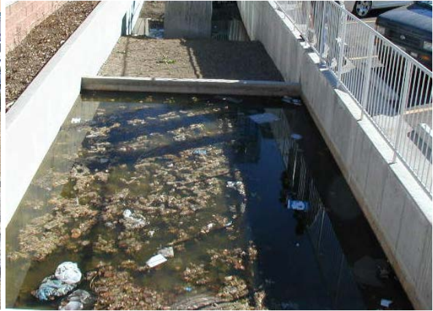
Photo 16. This detention facility is unattractive, difficult to maintain and, as a result, not maintained well.
