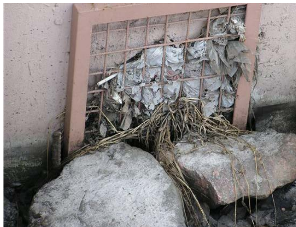
Photo 8. Trash rack on downstream end of pipe results in clogging and causes drainage and maintenance problems.
