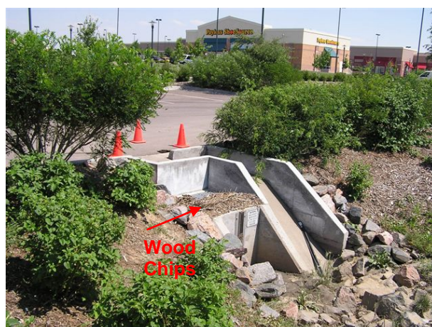
Photo 11. Curb and rundown provided to correct problem in Photo 10. However, wood chips should not have been placed in the basin, resulting in clogging of the outlet's trash rack.
