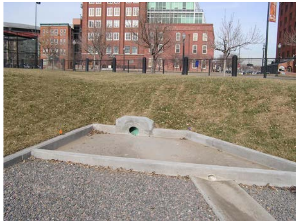
Photos 17 and 18 show a properly designed inlet, forebay, trickle channel and outlet in an urban setting that are easy to maintain and are well maintained.
