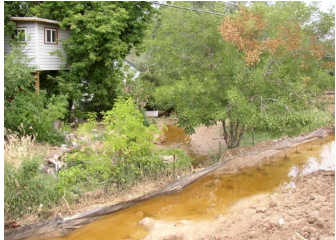
Photo 24. Silt fence must be properly installed and maintained to serve as an effective construction site BMP. Silt fence should be removed when final stabilization is achieved; otherwise it becomes construction trash left on a completed site.
