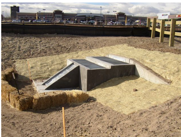
Photos 21 and 22 show before and after construction photos show how straw bales left on site can clog outlet structures later.
