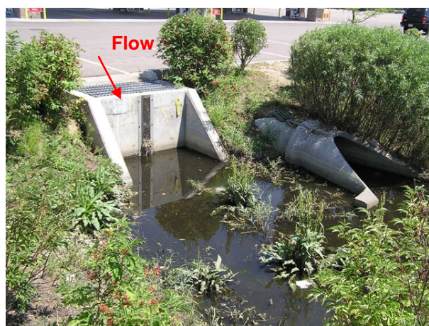
Photo 10. Flow from this parking lot bypasses water quality treatment. The inflow pipe is also too close to the outflow. Lack of micro-pool also caused outlet clogging and standing shallow water.
