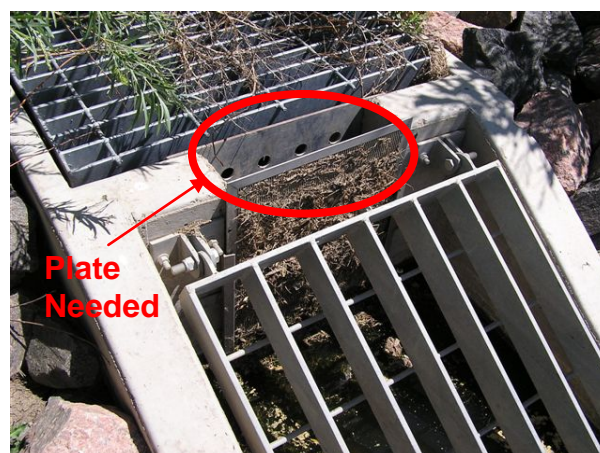
Photo 14. Clogged outlet structure. This structure needs a plate over the top to keep trash away from the orifices. A micro pool would also help to reduce this problem.
