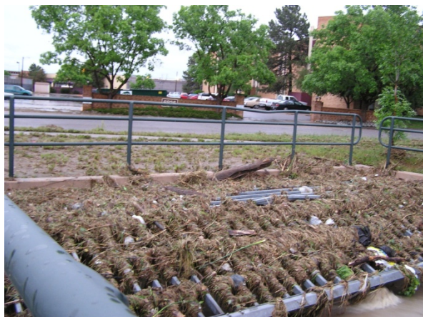
Photo 6. Debris blocking trash rack at culvert.
