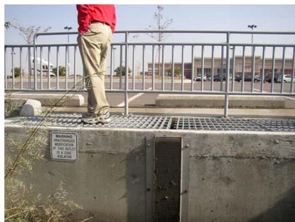
Photo 13. Flow from this parking lot bypasses water quality treatment basin's outlet and drains directly into the downstream vault.
