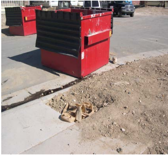
Photo 25. Improper waste disposal, especially with trash bin sitting in the gutter, is a source of construction site pollution. Oil, paints, concrete washout water, spill cleanup material and other potentially hazardous materials should be properly disposed of in designated receptacles and away from drainage facilities.
