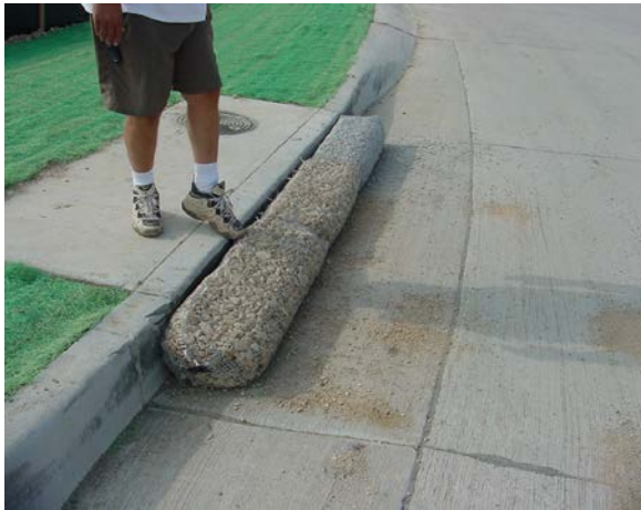
Photo 23. Inlet protection, a secondary line of defense commonly used on construction sites, must allow inlets to operate during larger runoff events. When inlet protection measures block inlets completely, street flooding and potential for flood damage is worsened, and nearby residents are more likely to attempt to remove the inlet protection to alleviate flooding, leading to uncontrolled sediment discharges to the storm sewer.
