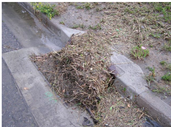
Photo 5. Debris blocking street inlet.
