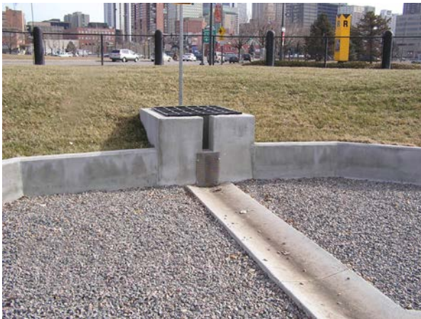
Photos 17 and 18 show a properly designed inlet, forebay, trickle channel and outlet in an urban setting that are easy to maintain and are well maintained.
