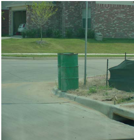
Photo 27. Containers should be labeled and stored in designated locations where potential spills can be controlled. Containers should not be stored near the flow lines or gutters, inlets or other watercourses on the site.
