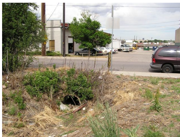
Photos 2 and 3 show a large box culvert to accommodate upstream development relative to a small downstream CMP, which may exacerbate flooding problems on the property downstream.
