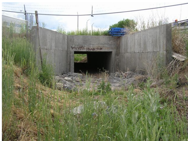
Photos 2 and 3 show a large box culvert to accommodate upstream development relative to a small downstream CMP, which may exacerbate flooding problems on the property downstream.
