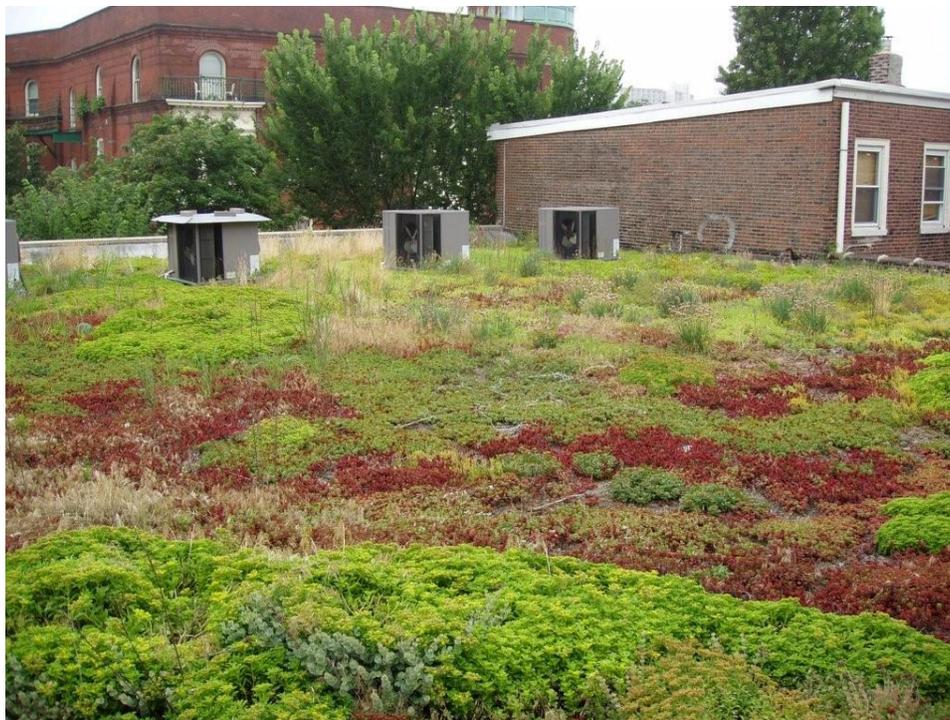
Figure 4-22. Example of Extensive Green Roof, Philadelphia, PA, Design Guidance (Source: UNHSC)
